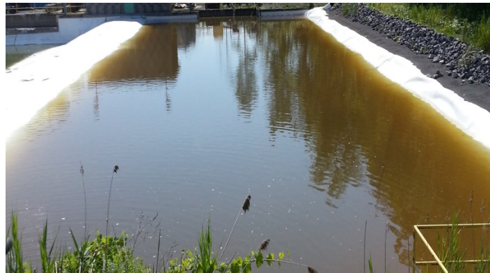
Figure 7 – Onsite Evaporation Pond (1 of 2 shown)
