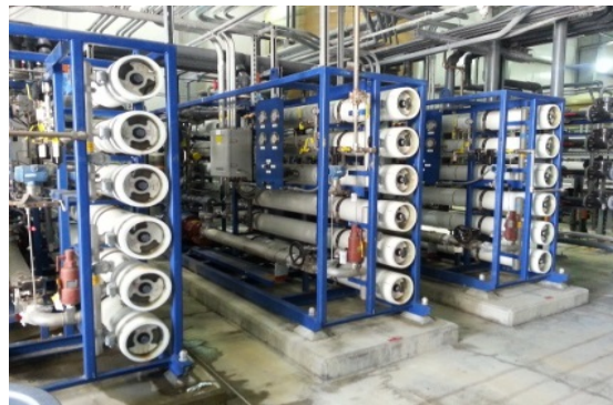
Figure 5 – RO Module Figure 6 – Brine Recycling RO Membrane System
