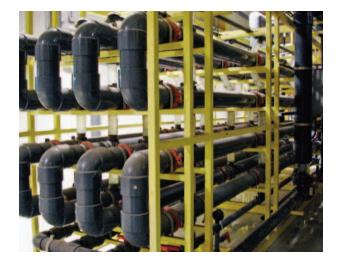
The 6 gallons of brine left will be four times more concentrated than the original 25 gallons, but by reducing the volume of brine by a significant amount, factories can reduce disposal costs and increase usable water production with the exact same volume of water they originally had coming through the doors, all while reducing their disposal footprint to more manageable levels.
