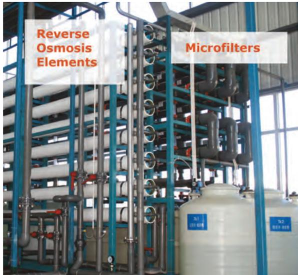
Low pressure Microfiltration has been around for decades as treatment for sewer discharge. Improvements in the membrane technology over the past decade have made MF/RO truly reliable for **recycling water with membrane life beyond 5 years.** These improvements also allow an industry to improve discharge reliability now while setting up for water recycle in the future and ultimately ZLD in the distant future as economics and the regulatory climate changes moving forward.
