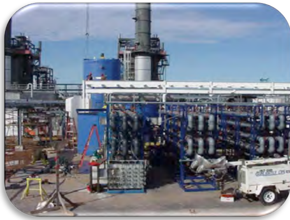
Figure 3 – DF Membrane System Installation
