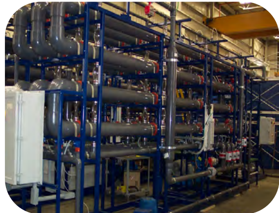
Figure 4 – DF Membrane Skid Assembly
